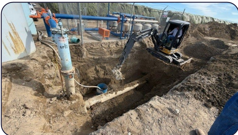
6P12 Leak Repair
