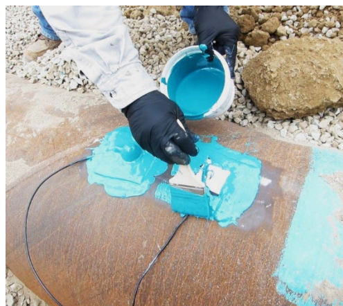
Sealing test station leads with epoxy
