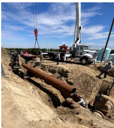
Moving steel pipe into position
